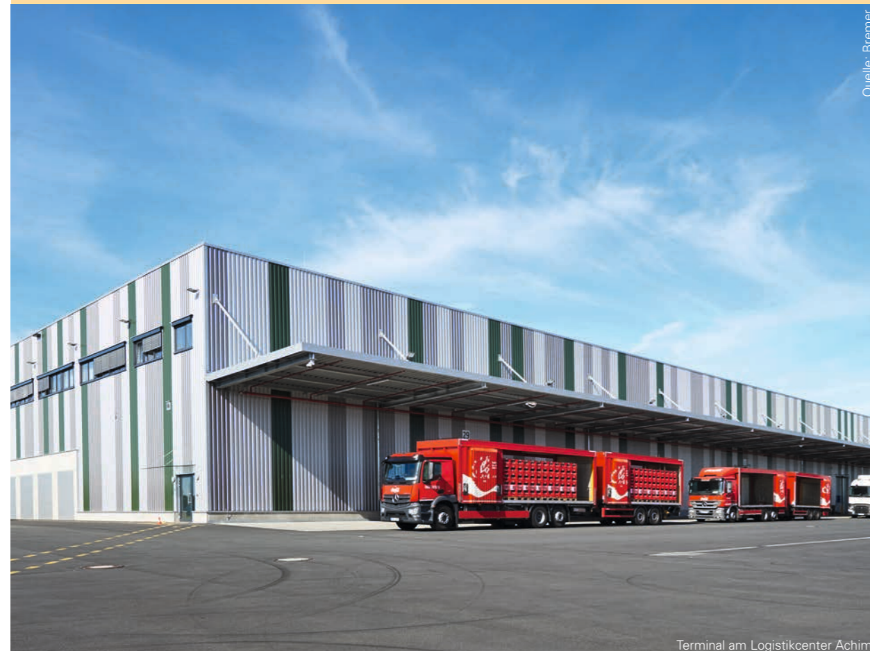
Terminal am Logistikcenter Achim
